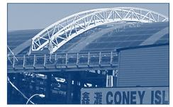
The newly reconstructed, subway station at Stillwell Avenue, Coney Island, Brooklyn is the city's first solar-powered train terminal. The station's 76,000-square foot stateof-the-art solar roof is expected to contribute approximately 250,000kilowatt hours a year to its nontraction power needs.
