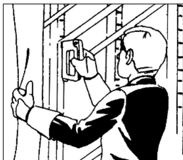
... and then cover with vapor barrier.
