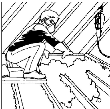
Before installing loose insulation, be sure to staple in a vapor barrier. Then, pour in the insulation and level it off.
