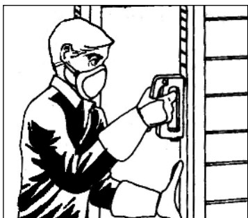
Insulating an exposed exterior wall: Staple insulation between studs ...
