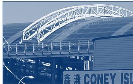
The newly reconstructed, subway station at Stillwell Avenue, Coney Island, Brooklyn is the city's first solar-powered train terminal. The station's 76,000-square foot state-of-the-art solar roof is expected to contribute approximately 250,000-kilowatt hours a year to its non-traction power needs.
